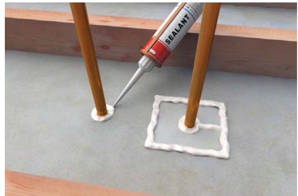
Figure 1: Sealing of Perforations Through Plasterboard Ceiling
